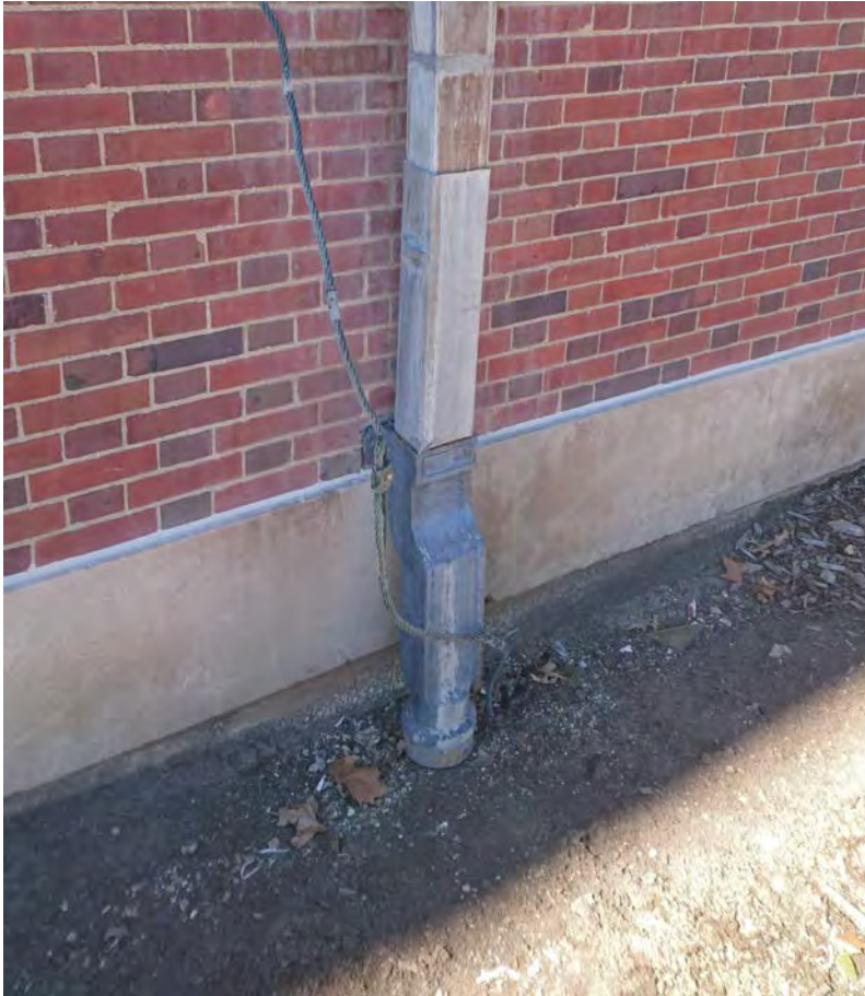
Figure 8: Typical downspout connection to storm drainage piping.
