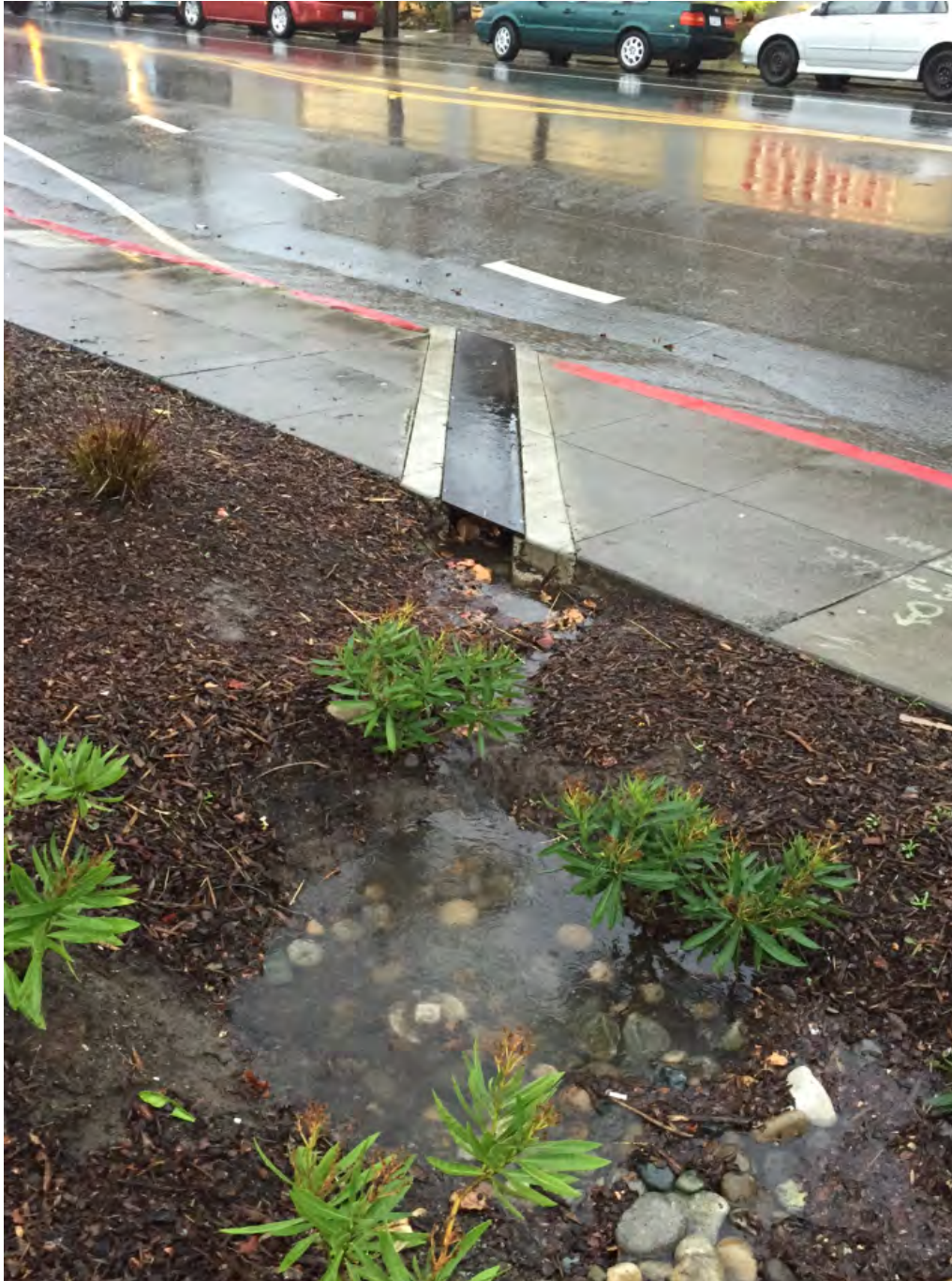
Figure 20: Example of stormwater runoff through a sidewalk. Image source: https://ruskinkhartley.com/tag/water-quality/#jp-carousel-1976
