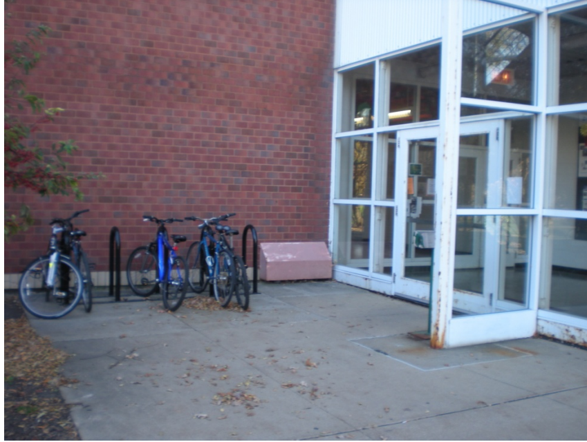
Agricultural Engineering Sciences Bldg 2
