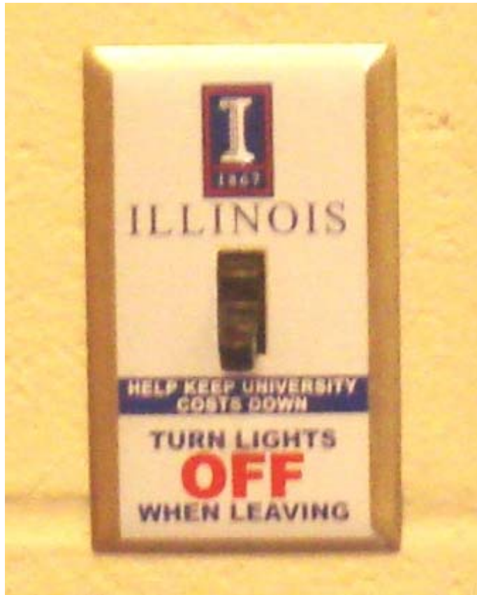
Typical Wall Switch to be replaced by
