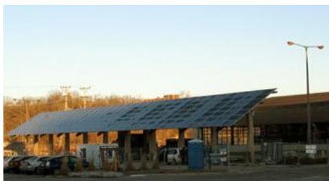
Figure 3 University of Iowa PV Station
