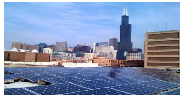
Figure 5 Lincoln Hall-UIC PV Array
