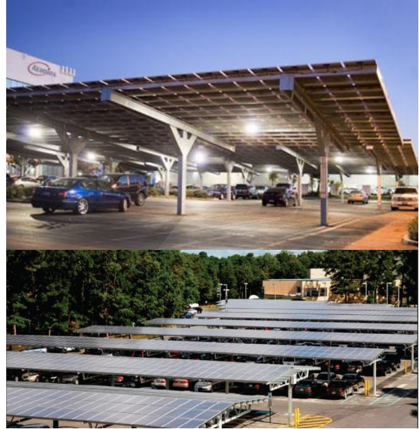
Figure 12. Solar Canopies for Open Parking Lots
