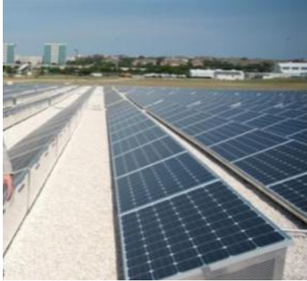
Figure 1 University of Texas PV Array
