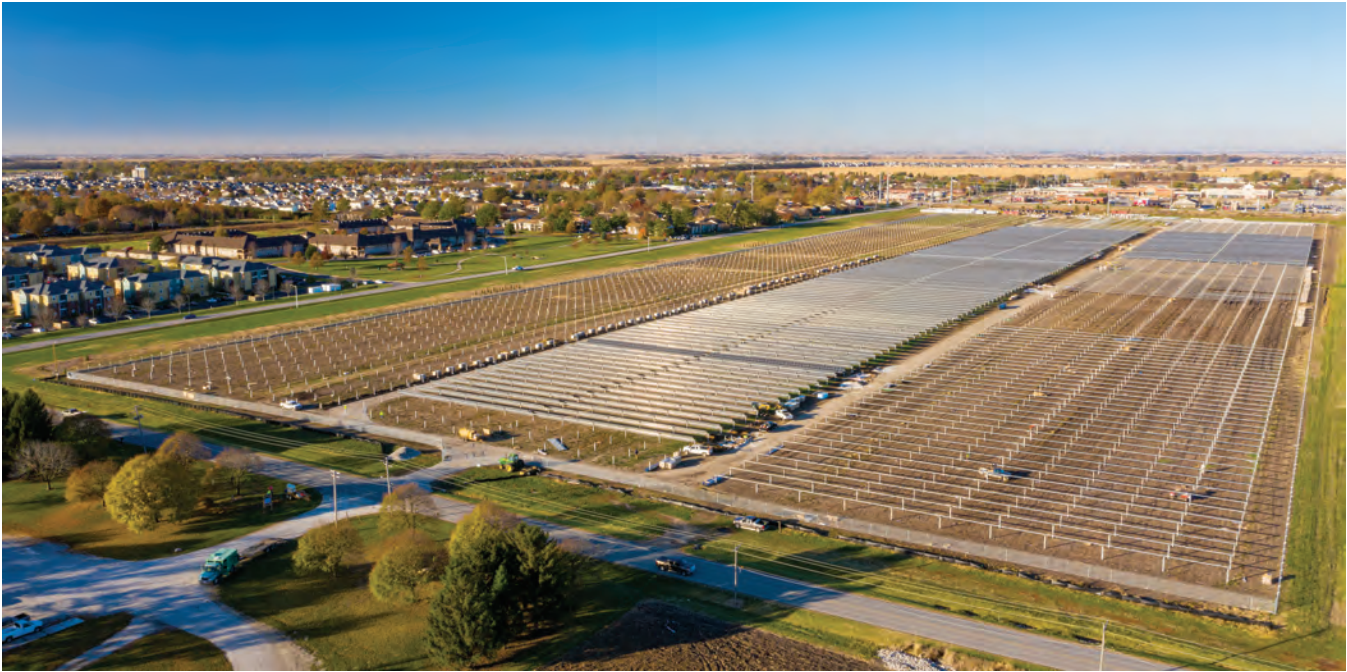
Solar Farm 2.0, a 12.32 megawatt (MWdc) utility-scale array located on campus.
