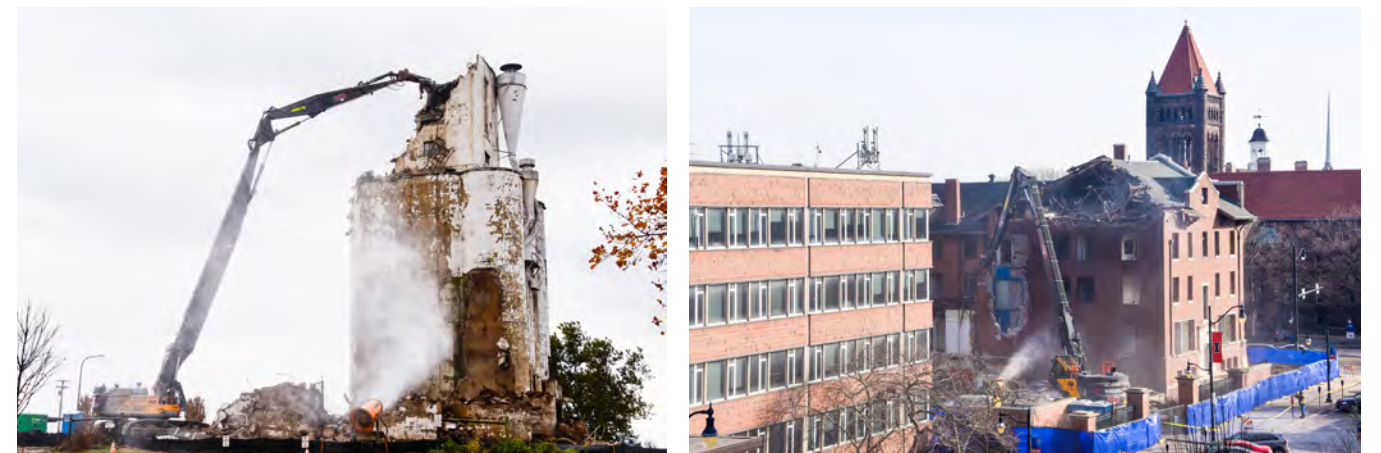
Building demolitions on campus. Building demolitions have a significant environmental impact because they result in the discarding of carbon-intensive building materials and drive demand for new, high-impact building materials.
