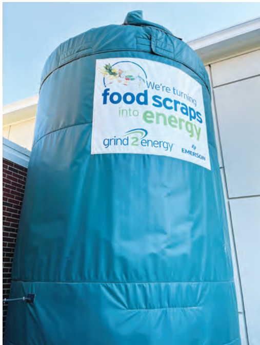
Above: The Grind2Energy system collects food waste from university dining halls so that it can be transported to the Urbana-Champaign Sanitary District and converted into energy. Below: A new, state-of-the-art baler machine was installed at the Waste Transfer Station in 2024 to enhance campus-wide recycling efficiency.
