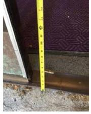
Figure 15 – High Threshold
