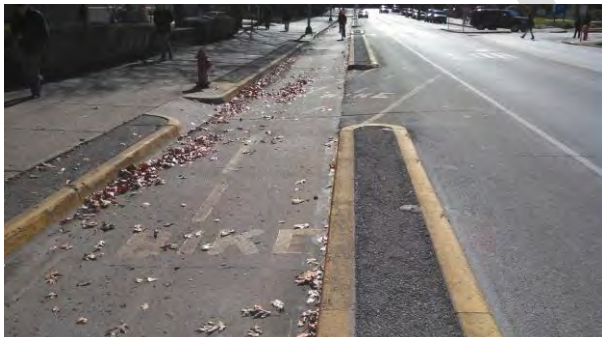
Inconsistent markings on Wright Street side path (#90) Photo by Geoff Merritt
