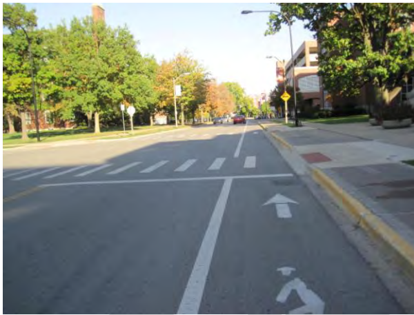
Existing Bike Lanes on Gregory Drive at Goodwin Avenue (#240). Note former side path along curb is still visible, to be fully removed as part of Phase 3. Photo by Holly Nelson
