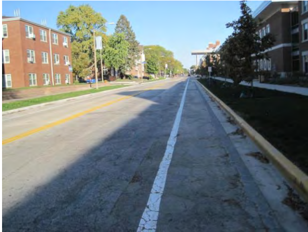
Existing Bike Lane on Gregory Drive near Ikenberry Commons (#240) Photo by Holly Nelson
