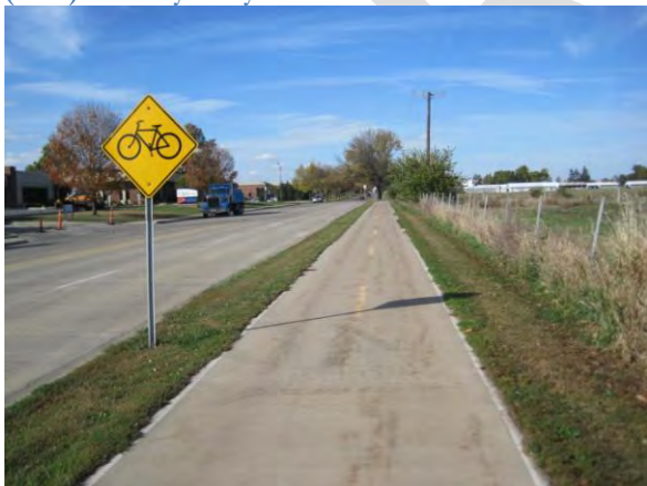
Shared Use Side Path along First Street south of Kirby Avenue (#480) Photo by Holly Nelson
