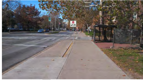
Green Street at Mathews Avenue, where existing side path goes through a bus stop. (#150) Photo by Geoff Merritt
