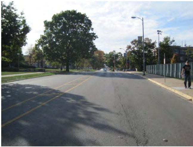
Pennsylvania Avenue (#300) Photo by Holly Nelson
