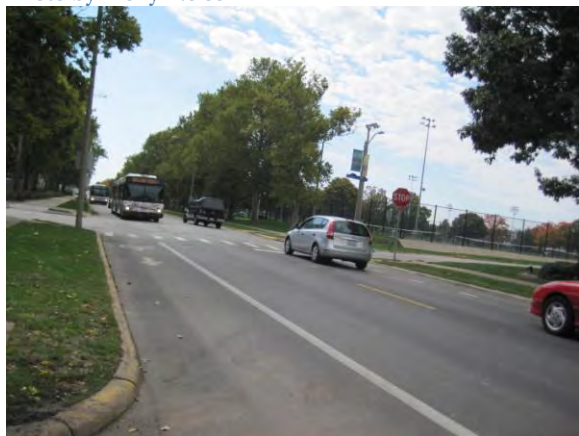
Existing Bike Lanes on First Street north of Gregory Drive (#670) Photo by Holly Nelson
