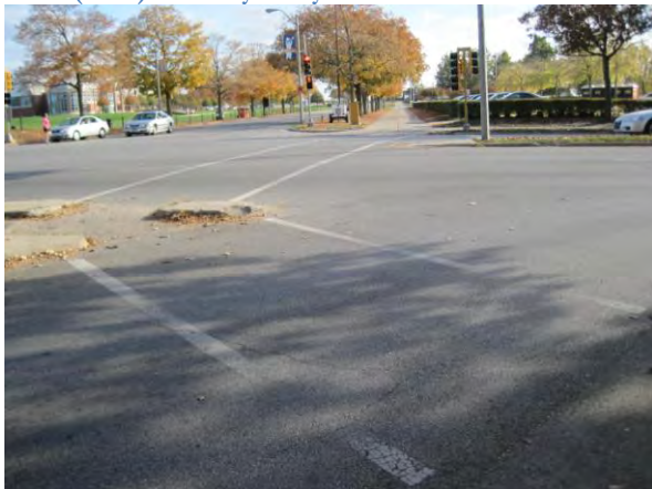
Pedestrian Crossing at Kirby Avenue (#390) and Fourth Street (#260/440) Photo by Holly Nelson
