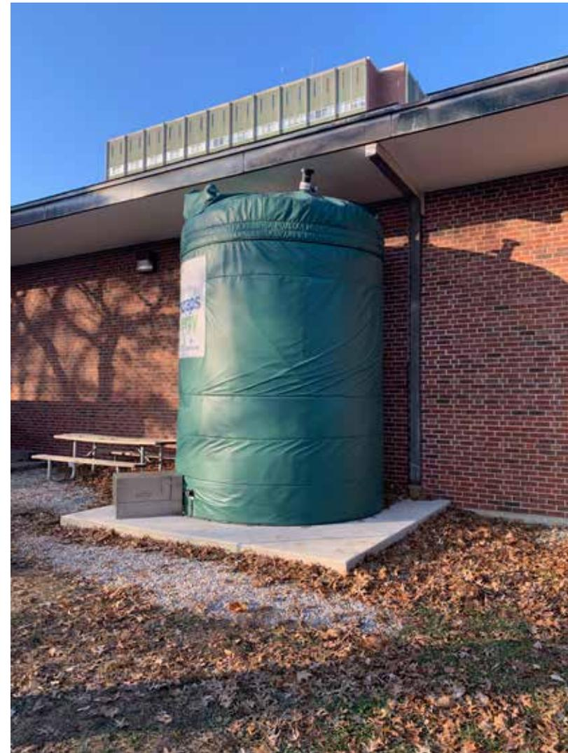
Ground dining hall food waste is emptied into the Grind2Energy holding tank (pictured). The slurry is transported to the Urbana-Champaign Sanitary District's anaerobic digester for electricity production.
