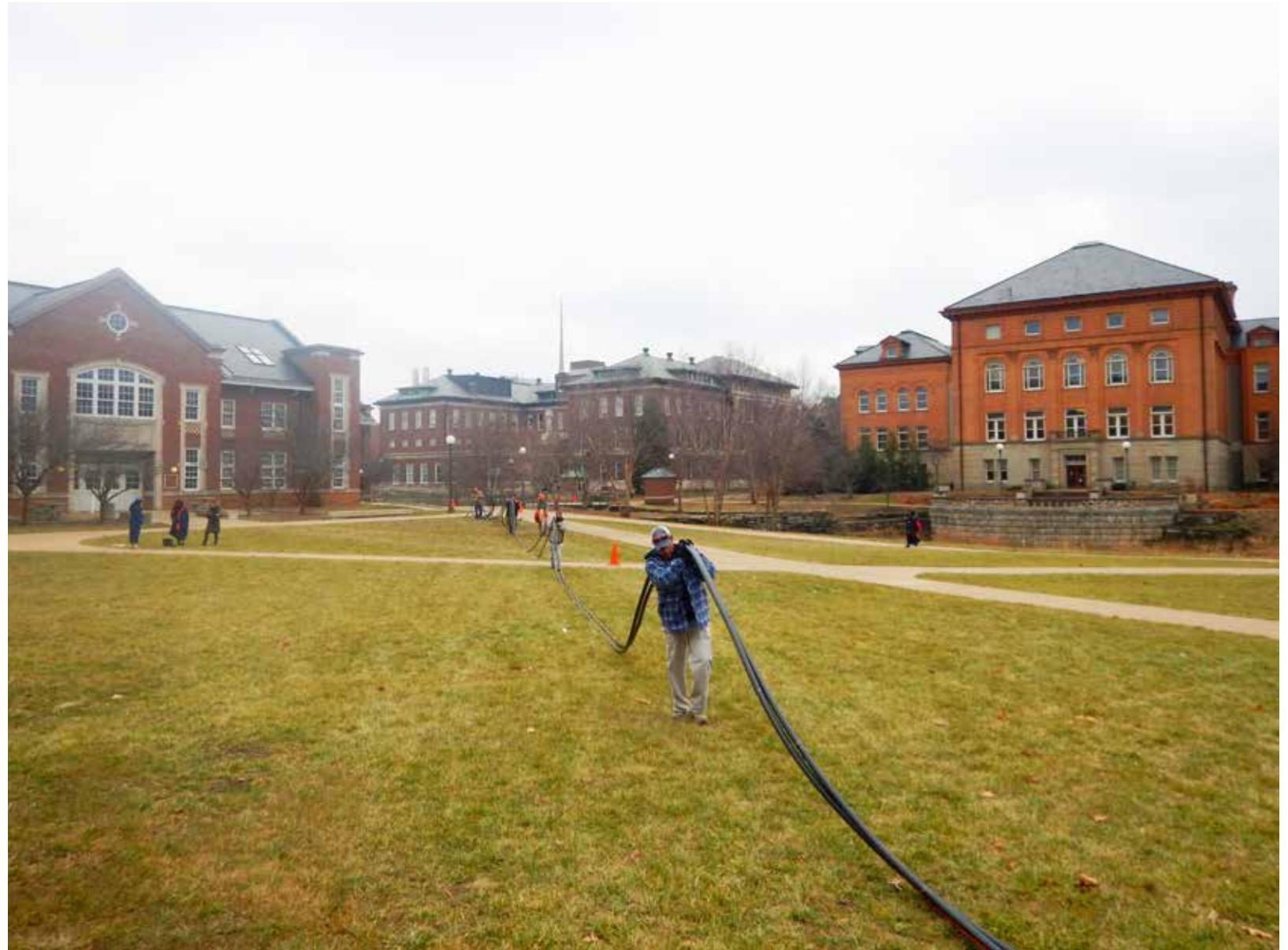
Geothermal loop and fiber optic cable installation on the Bardeen Quad, December 2018.
