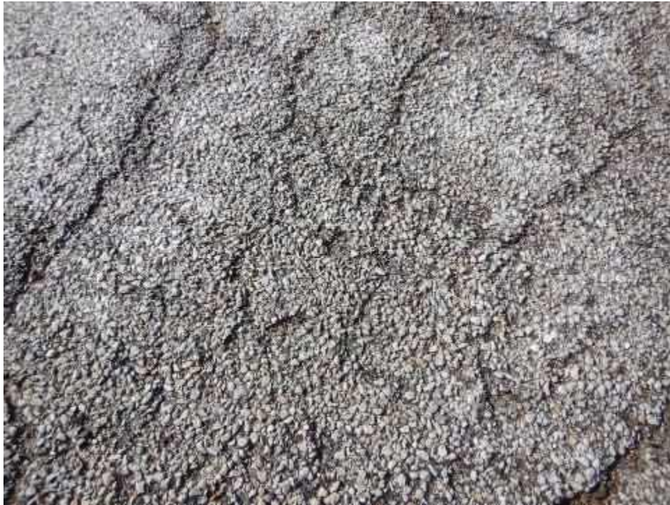
KIRKD-S20B-Raveling-(Sample Unit No. 01)
