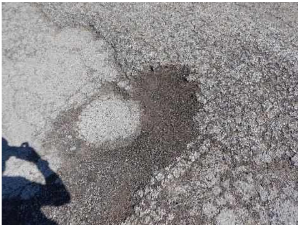
PEABYD-E06A-Raveling-(Sample Unit No. 01)
