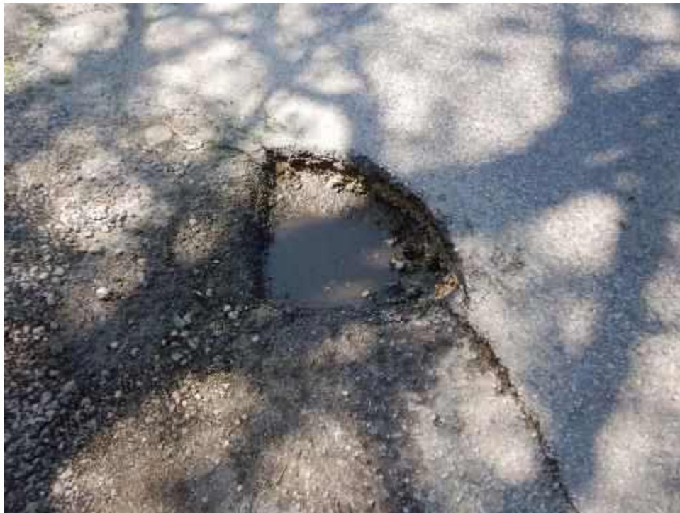
GOODWINA-US17-Pothole-(Sample Unit No. 01)
