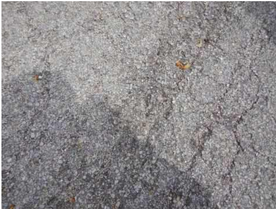
PENSYA-UW09B-Raveling-(Sample Unit No. 01)
