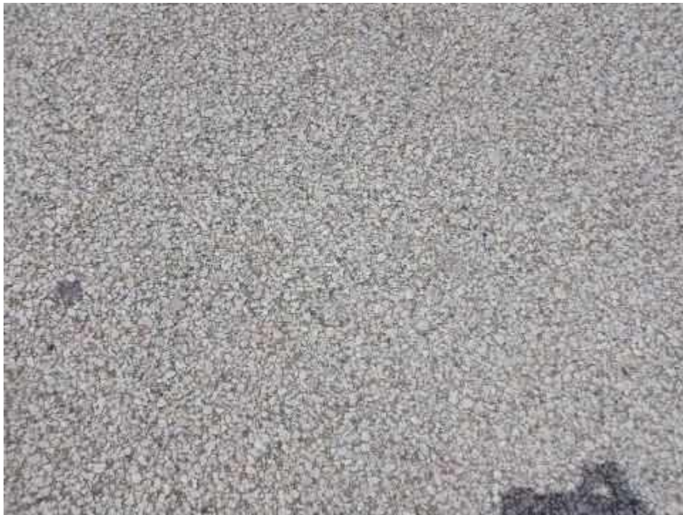
VRGNADR-US14A-Weathering-(Sample Unit No. 01)
