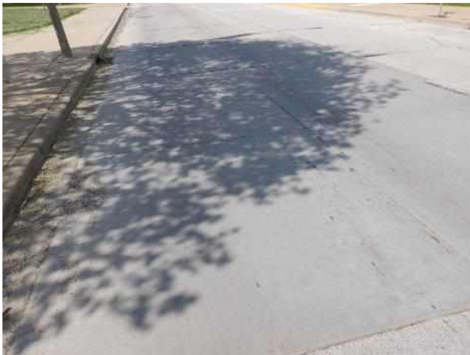
DORNRDR-US11BW-Patching-(Sample Unit No. 01)
