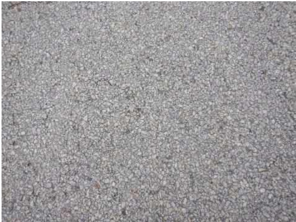
COLAGCT-UW09DN-Weathering-(Sample Unit No. 01)
