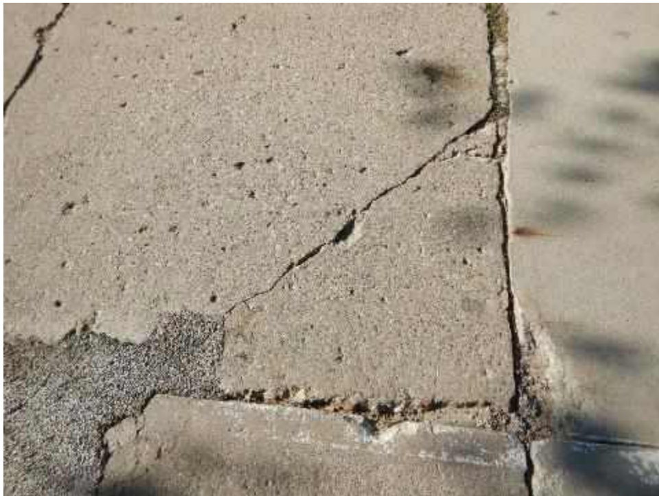
STMARR-E00B-Corner Break-(Sample Unit No. 01)
