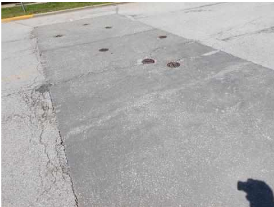
PEABYD-E01A-Patching-(Sample Unit No. 02)
