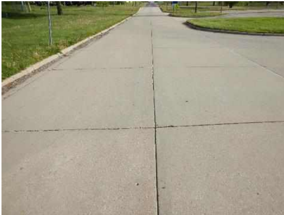
GRIFFITHD-S22B-Overview-(Sample Unit No. 01)
