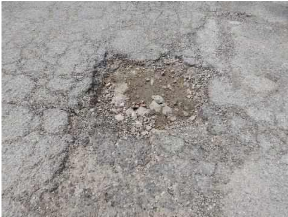
PENSYA-UW09A-Pothole-(Sample Unit No. 01)
