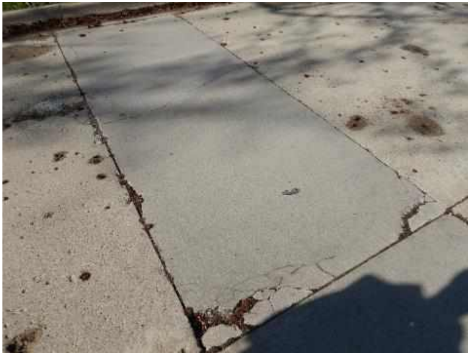
GERTYD-E00B-Large Patching-(Sample Unit No. 01)
