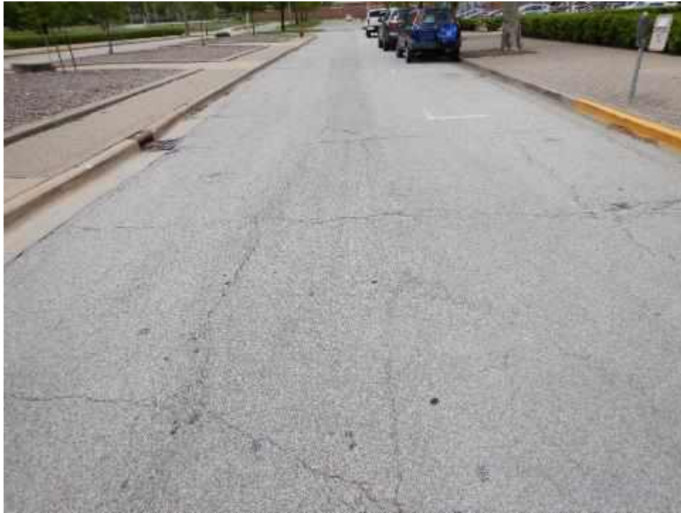
COLAGCT-UW09BN-Overview-(Sample Unit No. 01)
