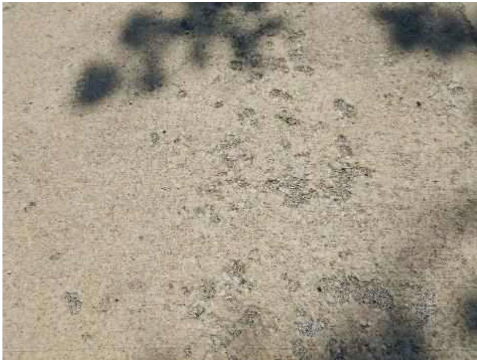
HAZELWDD-UW09-Scaling-(Sample Unit No. 01)
