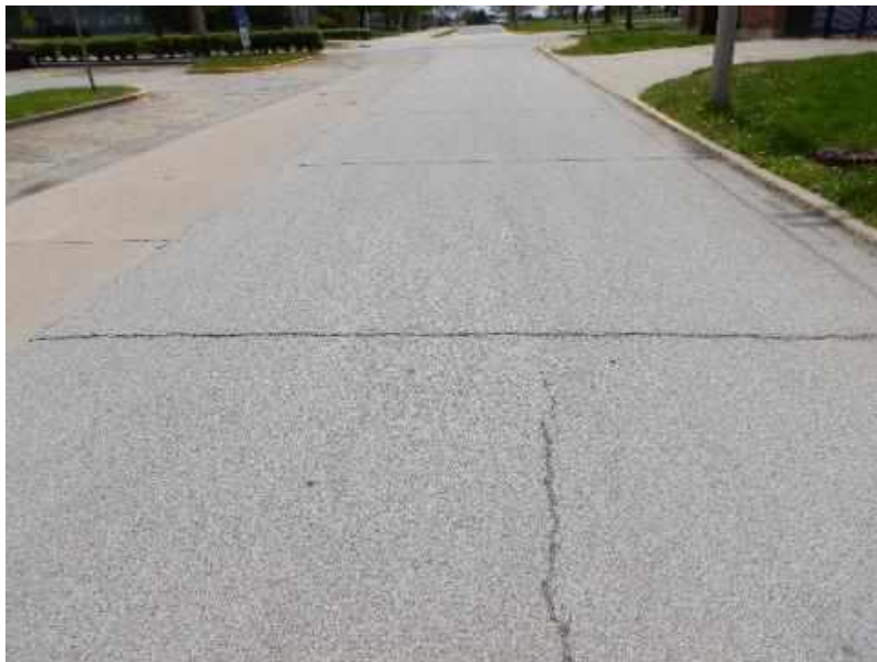
VRGNADR-US14BW-Overview-(Sample Unit No. 01)
