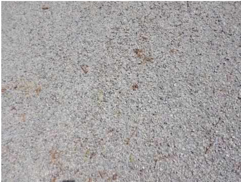
COLAGCT-UW09CS-Raveling-(Sample Unit No. 01)
