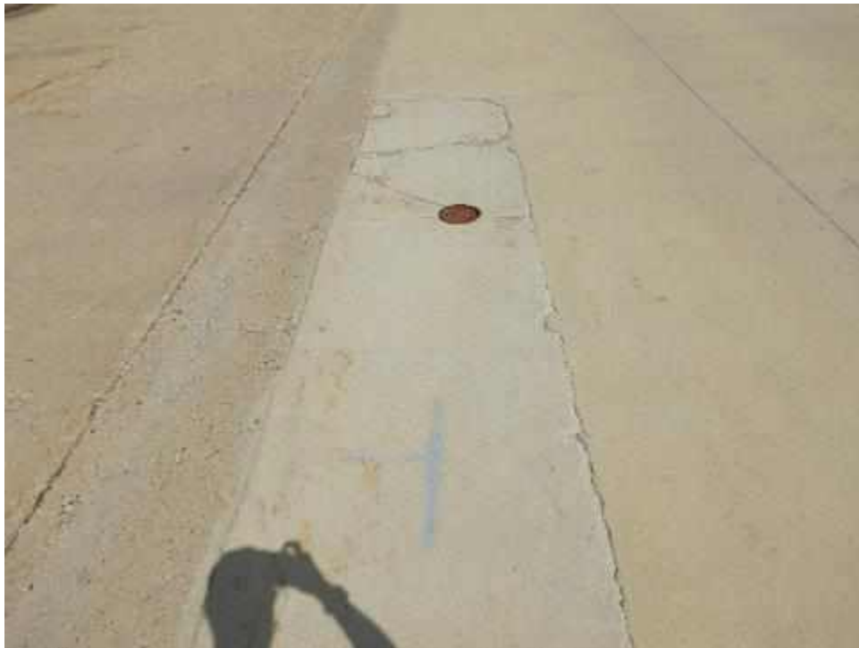
PEABYD-UW11-Large Patching-(Sample Unit No. 01)
