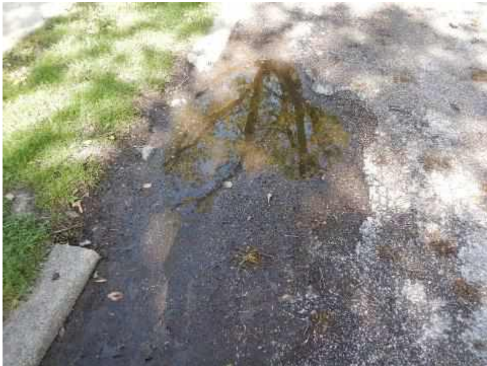
PEABYD-E06B-Depression-(Sample Unit No. 01)
