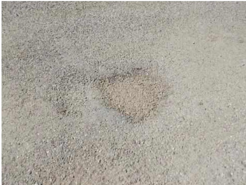
HAZELWDD-UW12A-Raveling-(Sample Unit No. 01)
