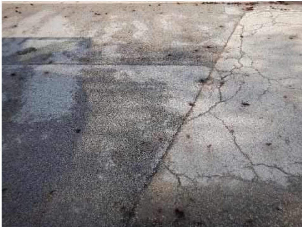
BAILEYD-E00-Patching-(Sample Unit No. 02)
