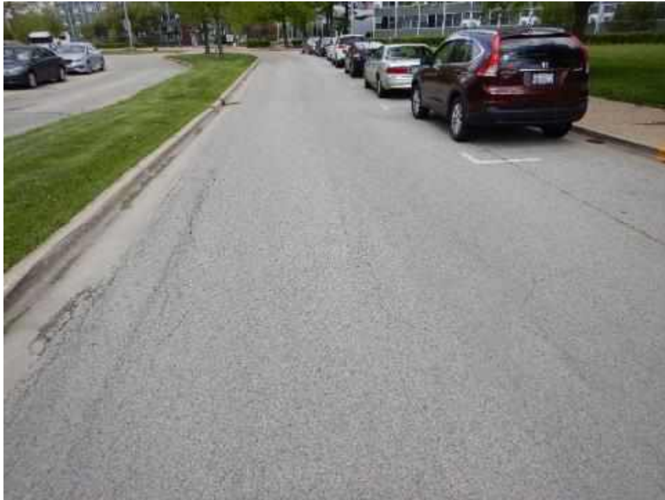
COLAGCT-UW09DN-Overview-(Sample Unit No. 01)
