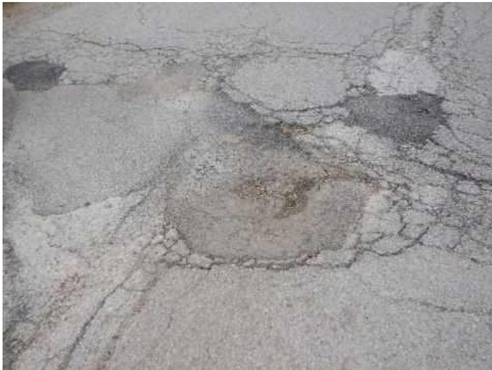
PENSYA-UW11A-Pothole-(Sample Unit No. 01)
