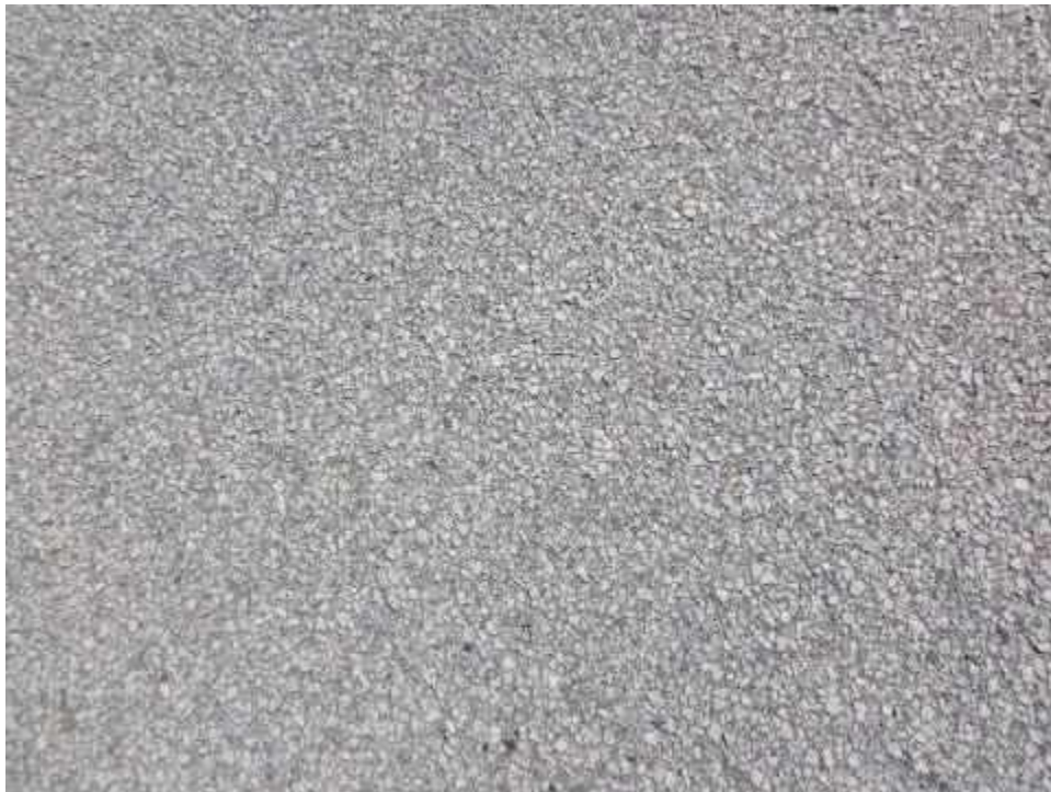
DORNRDR-US13E-Weathering-(Sample Unit No. 01)
