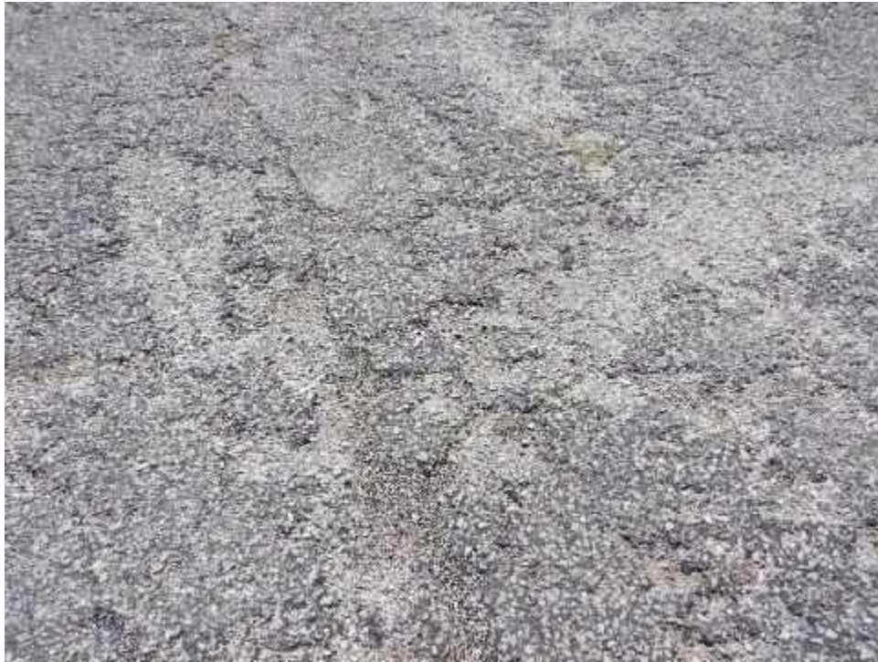
GOODWINA-US19-Raveling-(Sample Unit No. 02)
