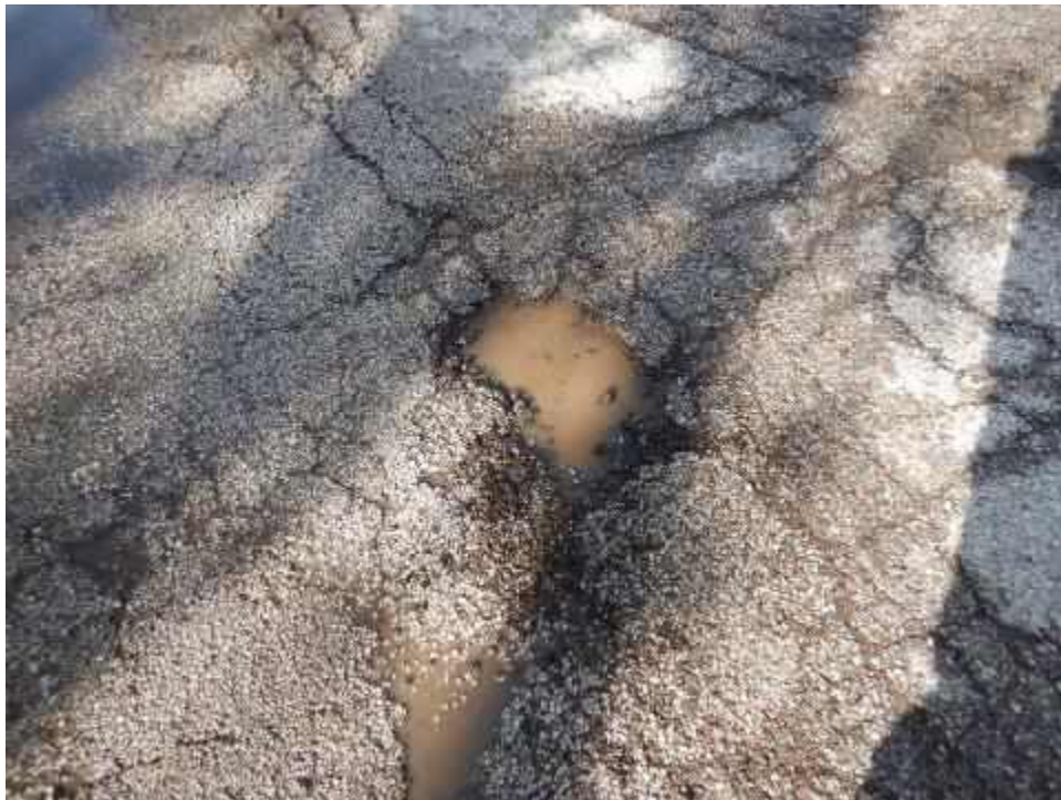
KIRKD-S20B-Pothole-(Sample Unit No. 01)
