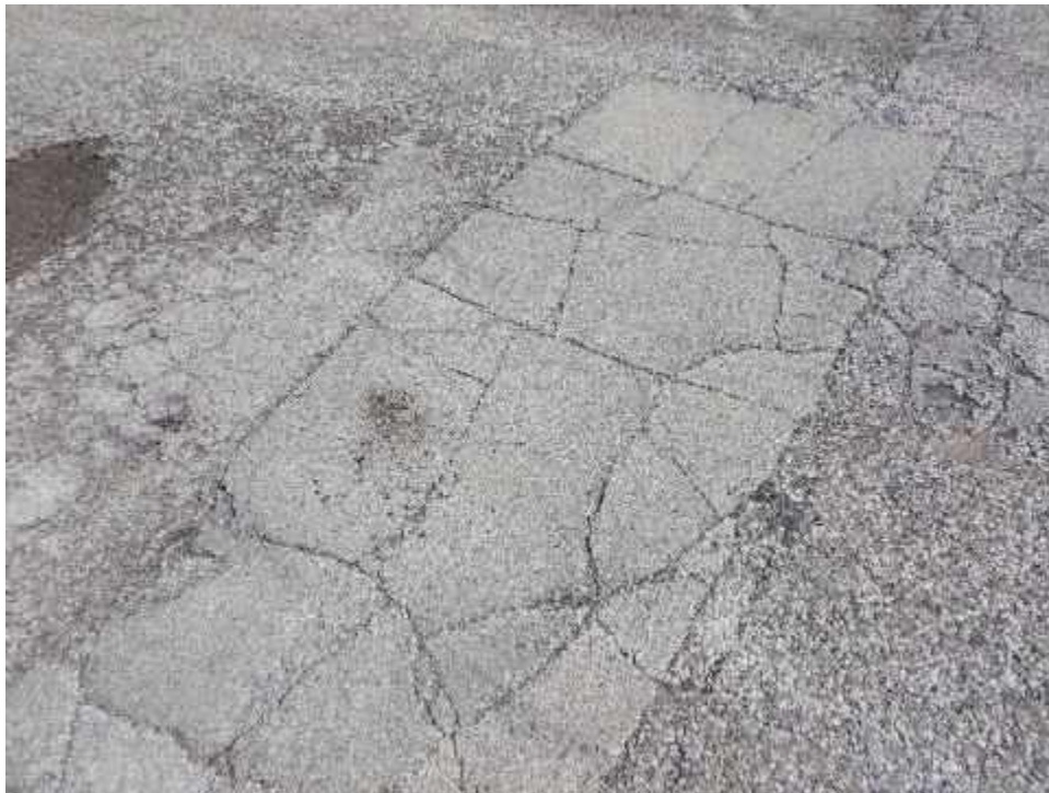
PEABYD-E06A-Patching-(Sample Unit No. 01)
