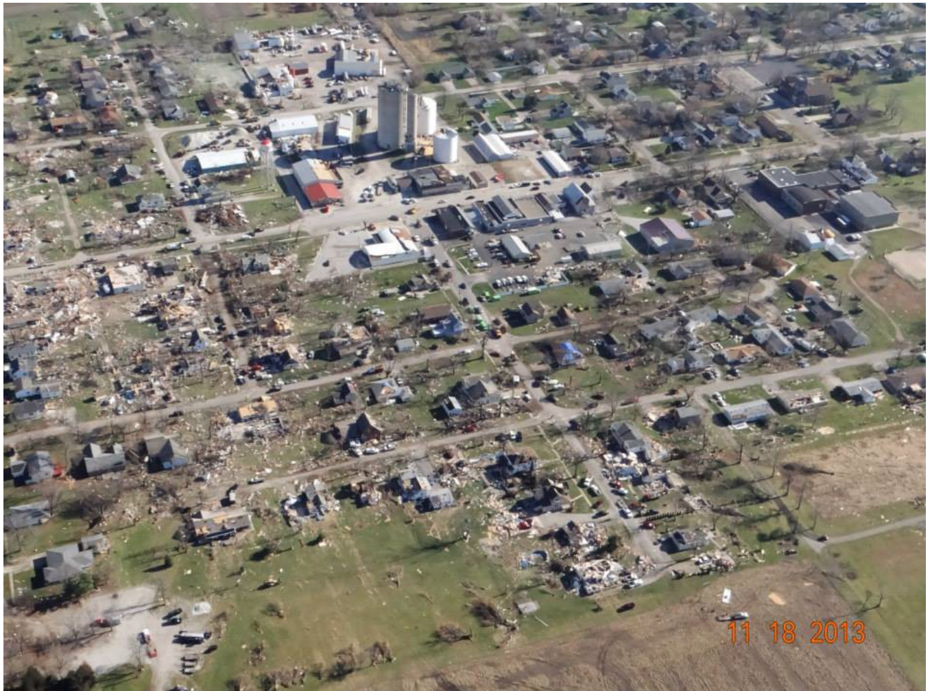
Figure 4-7. Damage to Gifford by EF-3 Tornado, November 18, 2013 Photograph
