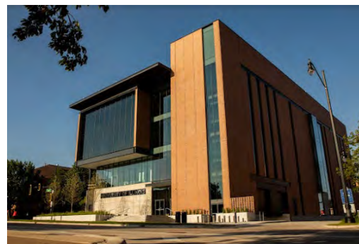
Campus Instructional Facility (CIF)
