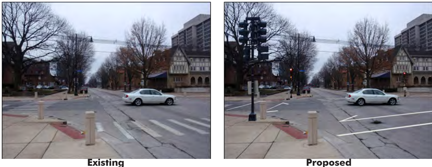
Figure 4.14: Existing and Proposed Traffic Controls at the Fourth Street/ Armory Avenue Intersection
