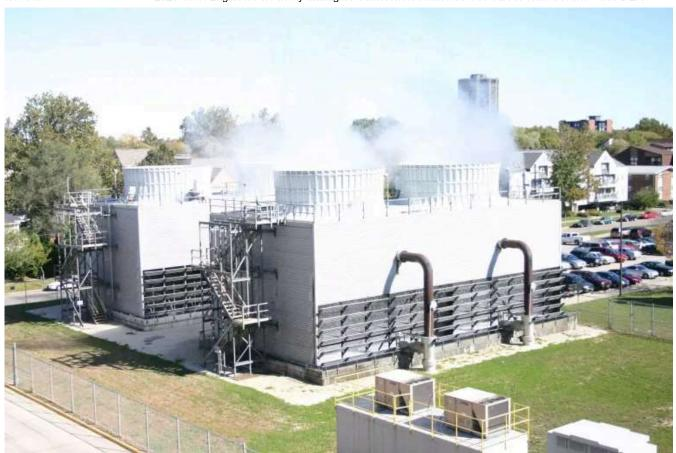
In 2004, a \$50M conversion to an alternative chilled-water configuration using regional chilled-water plants serving a large central-piping loop connecting campus buildings was started. The loop has reduced cooling energy consumption by an estimated 20 percent.
