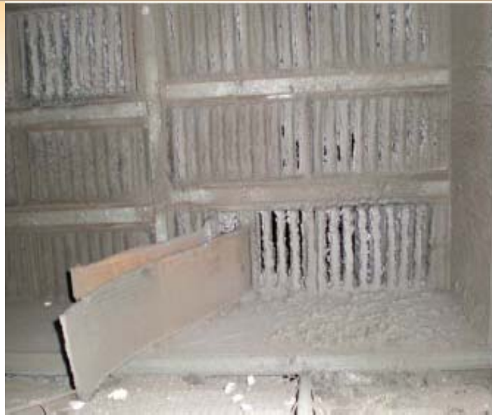
Air Silencer at Festival Theatre return air ductwork caked with dust
