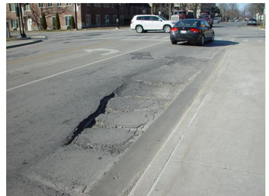
Wright Street Existing Pavement Condition
