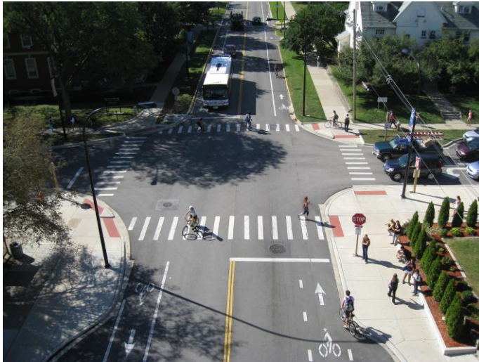
Goodwin Avenue & Nevada Avenue Complete Street on University of Illinois Campus
