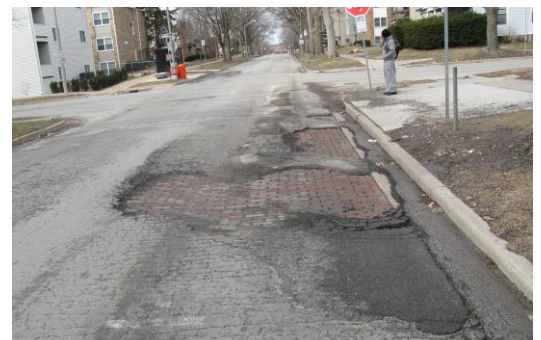
White Street Existing Pavement Condition
