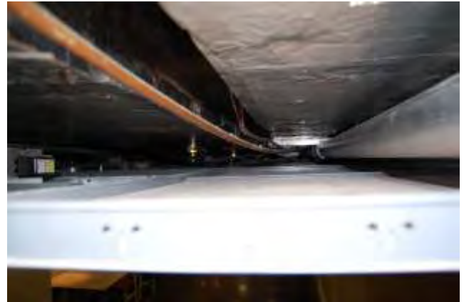
Looking East in the ceiling above corridor just south of the main kitchen.
