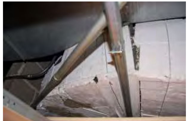
Asbestos insulated grease duct above main kitchen.
