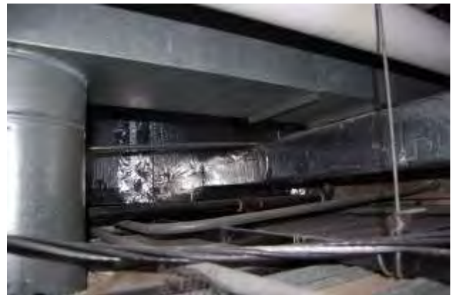
Looking South in the ceiling above corridor just East of the main kitchen.
