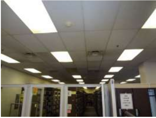
Approx. 10% of general lighting is connected to Emergency circuit
