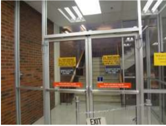
Door security system
