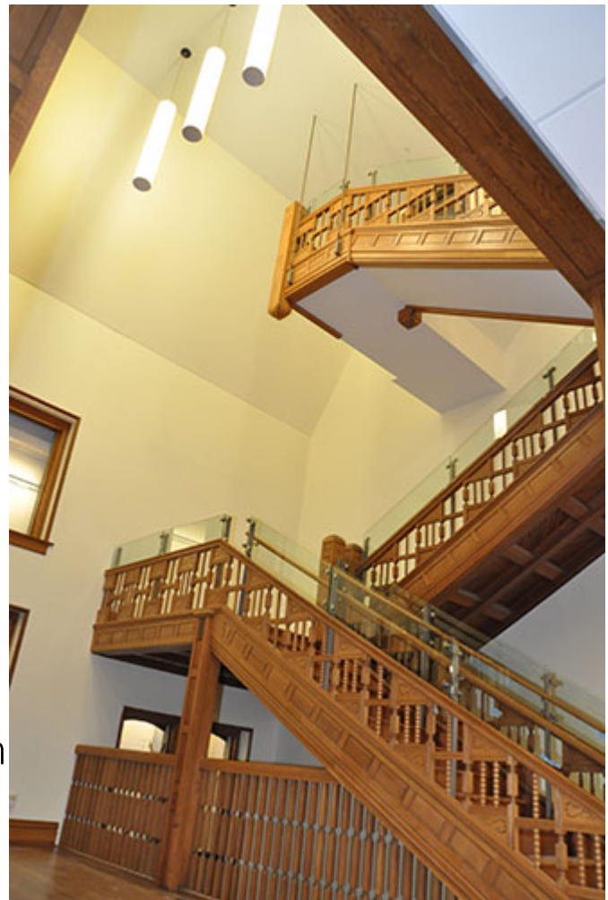
Part of the Natural History Building's LEED Gold certification came from the reuse of old materials, such as a portion of the wood used to renovate this stairwell on the north end of the building. (Photo by Heather Gillett.)
