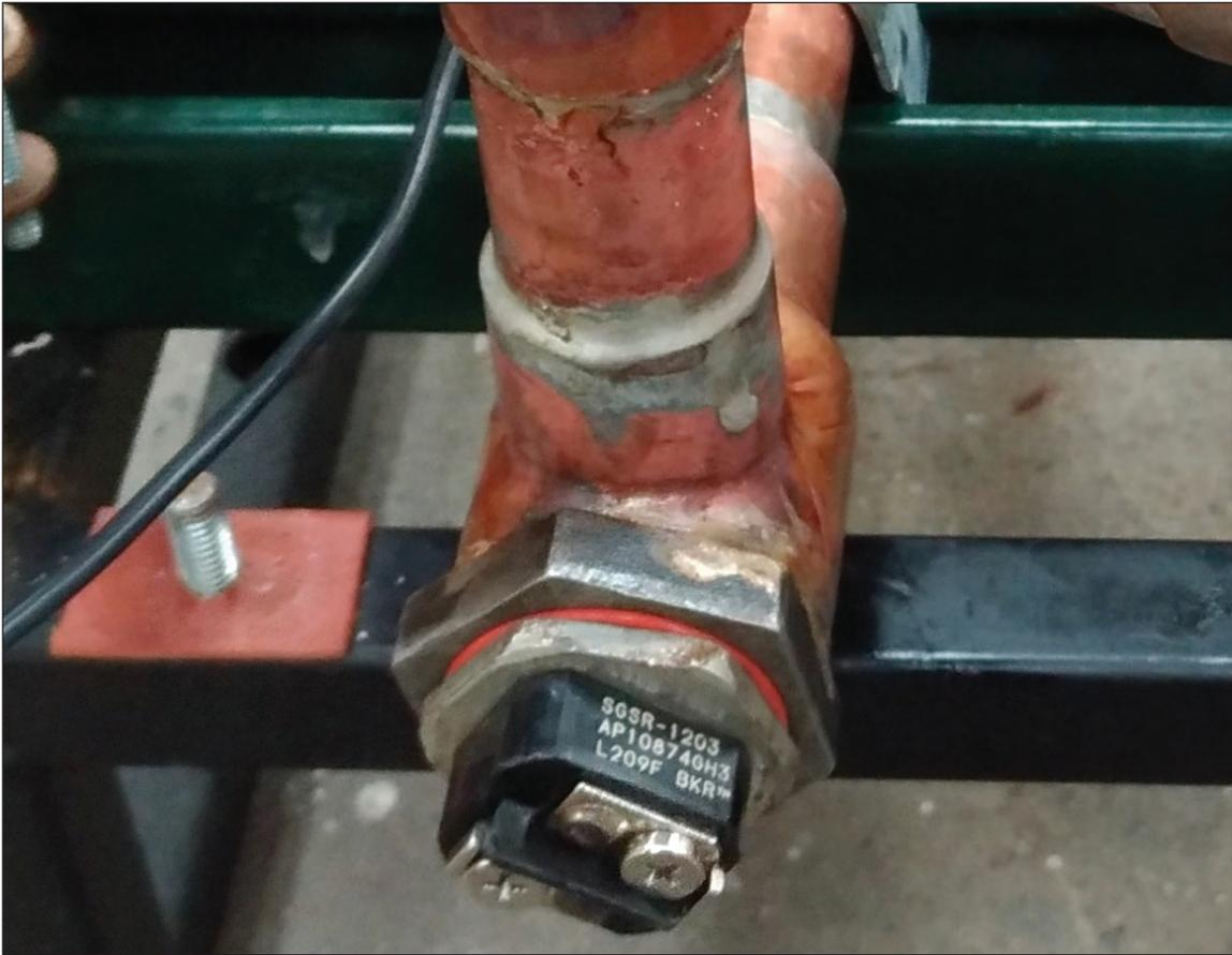
**Figure 6** The SGSR-1203 AP10874GH3 water heater element, labeled D in Figure 2.
