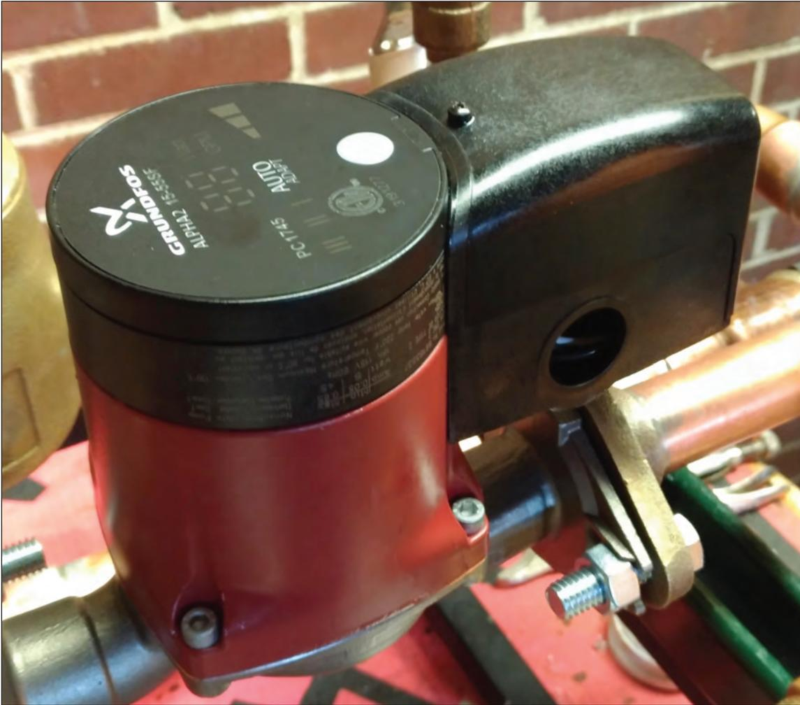
**Figure 9** The Grundfos ALPHA2 multispeed pump used to control the flow rate through the loop, labeled E in Figure 2. The pump can withstand extreme conditions in the heating system.
