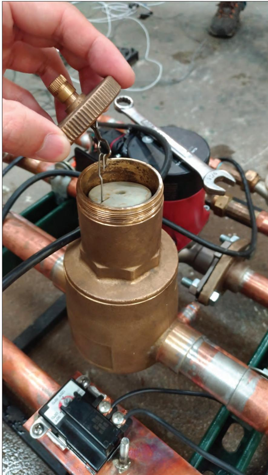
**Figure 5** Detail of the air eliminator with the floater inside, labeled B in Figure 2.
