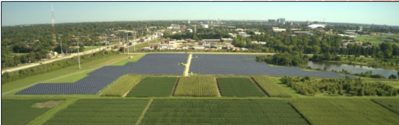
Solar Farm 1.0 (5 MW → 7,000 MWh/yr)
