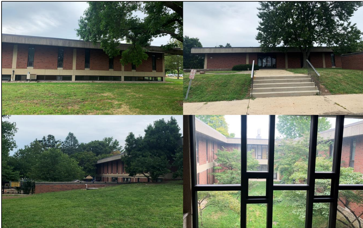
Figure 2 Exterior and courtyard of Children's Research Center
