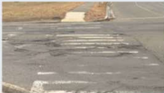
Faded crosswalk markings
