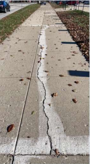
Cracks- more than 4 feet of accessible sidewalk (Count: 311)
