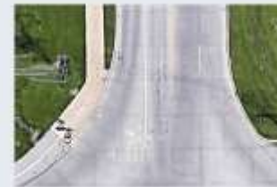
Lack of curb cuts and detectable warning details
