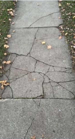
Cracks- more than 4 feet of accessible sidewalk (Count: 350)
