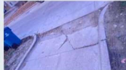
Driveway apron has maintenance issues
