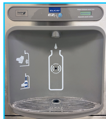
HYDRATION STATION EQUIPPED WITH BOTTLE FILLER
