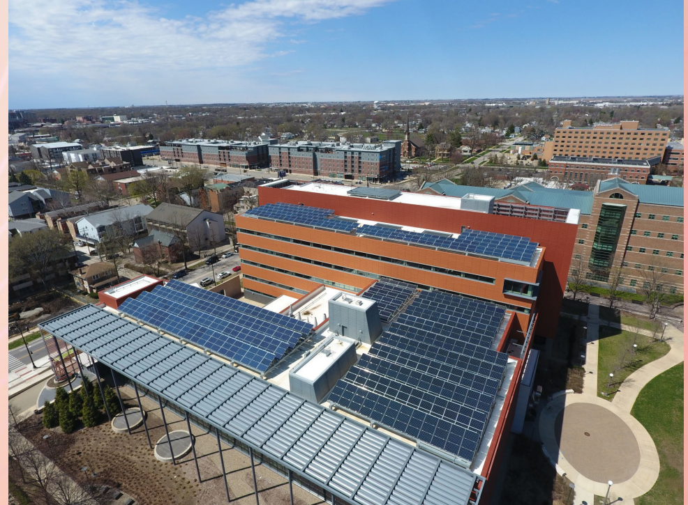
Electrical and Computer Engineering Building Rooftop Solar drone image 2019, courtesy of ECE department
