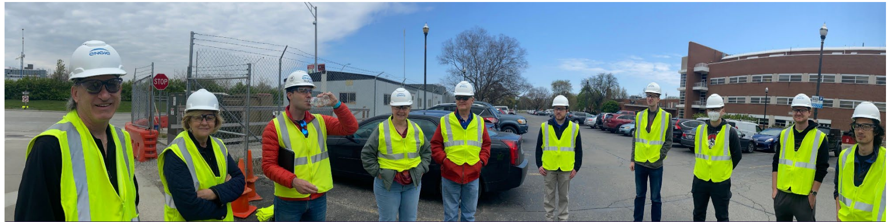
Hosted Construction Site tour for the College of Engineering's College Committee on Academic Affairs and CORE Teaching and Learning for College of Engineering teams.
