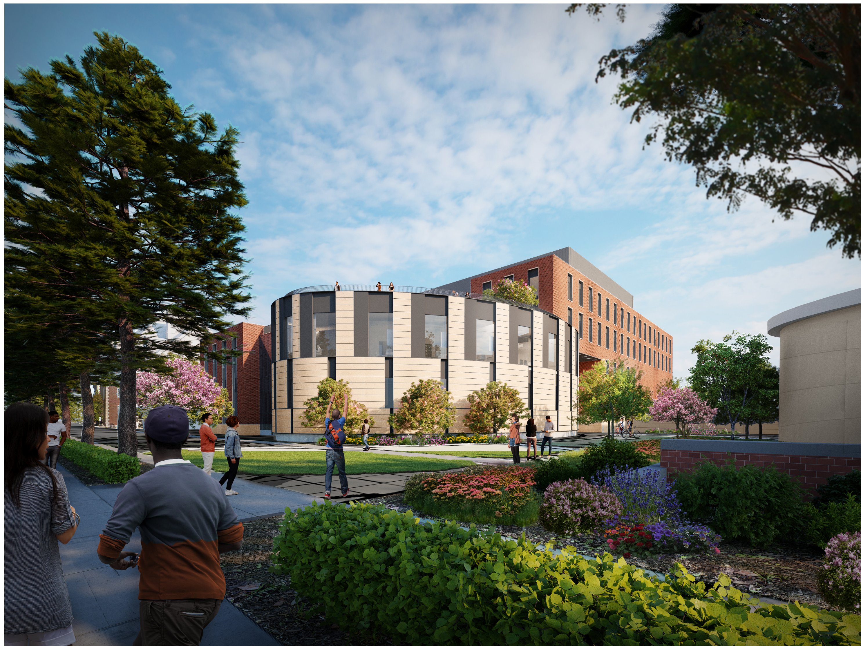
South view looking north
