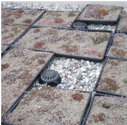
Green Grid System Weeks After Installation
