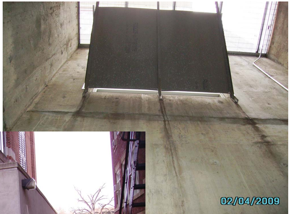
Photo 4: Existing shroud at relief air louver
