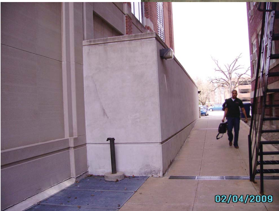
Photo 5: Exterior view of area well.
