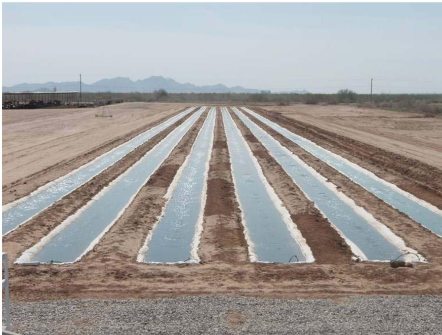
**Figure 3.** Outdoor ponds used at XL Renewables pilot plant in Vicksburg, Arizona. The troughs are constructed using traditional agricultural equipment and the bed liner provides aeration for growth.
