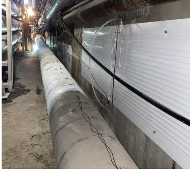
Figure 17. Panel Array Installed in Steam Tunnel
