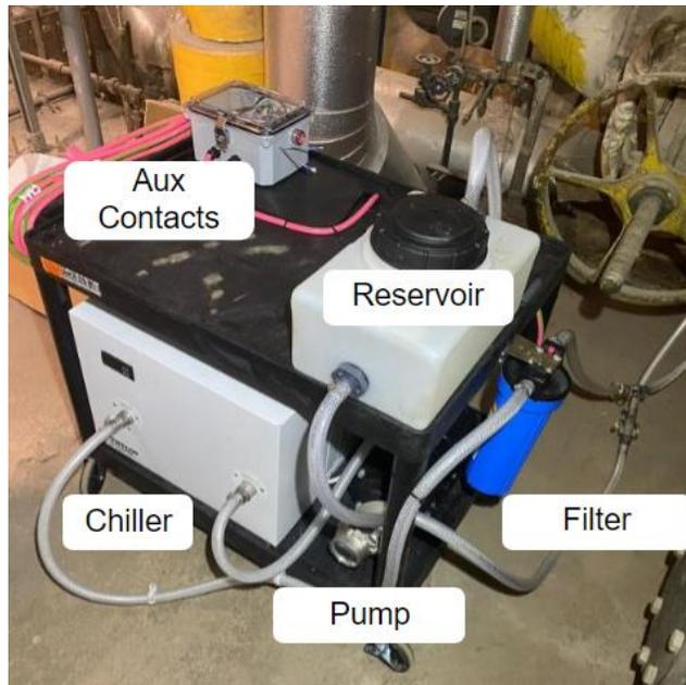
Figure 18. Cart for Component Housing Outside of Tunnel
