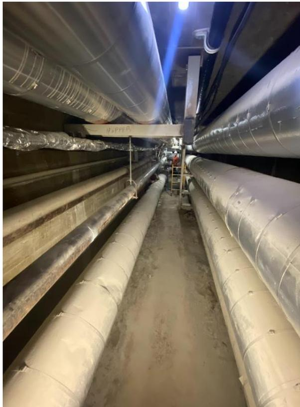
Figure 4. Steam tunnels at Abbott Power Plant
