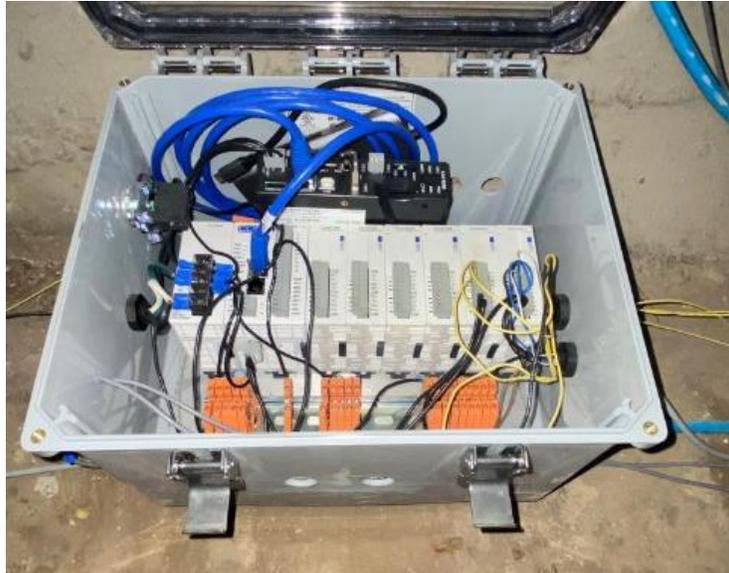
Figure 20. PLC and HMI Setup in Electrical Box
