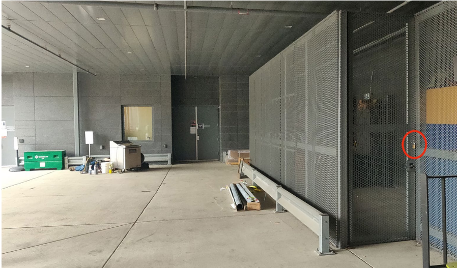
Entrance to cage from ECEB loading dock (facing north) Locked cage door is front right (lock is circled in red).
