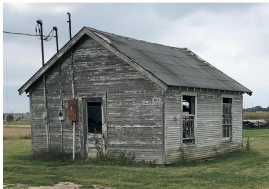
Building 931 (first building to have CornCrete installed)
