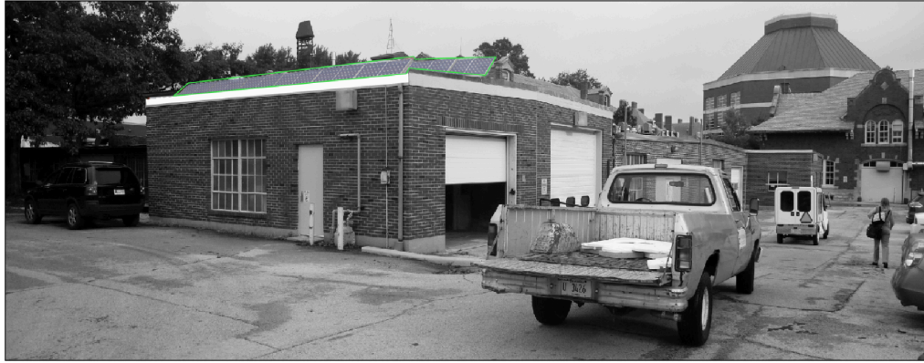
Visual Representation of solar panels installed on the roof of building #18 (garage at south east corner). By Tingting Peng (Arch 576 - Fall 2014)
